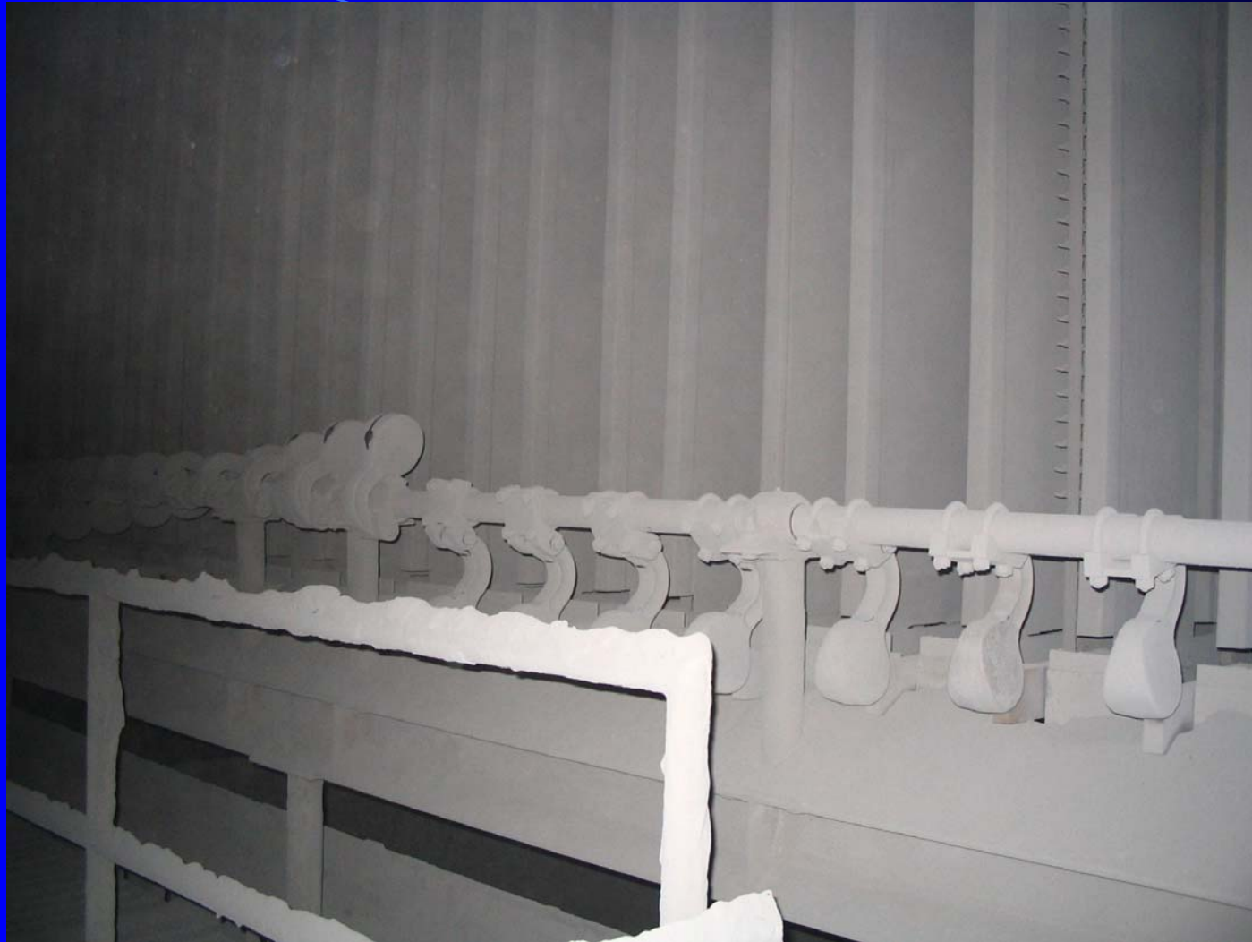
Rotating Hammer Rapping System
